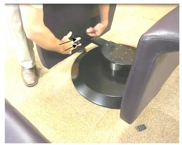
2. Tracks slide onto Shoe during re-assembly
