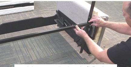
Install the Square Back Tube with 7/16" socket and wrench – Tube mounts on **TOP** of bracket
